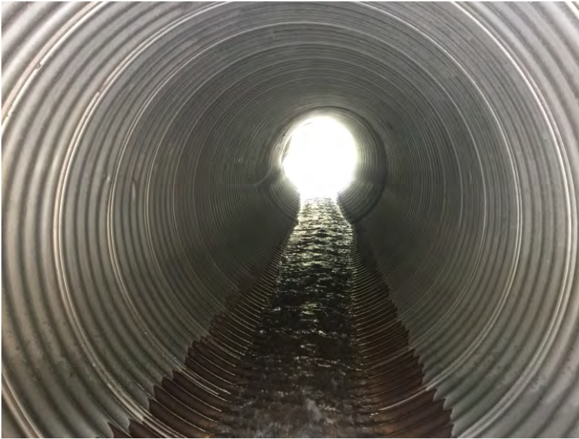
Looking through culvert from inlet
